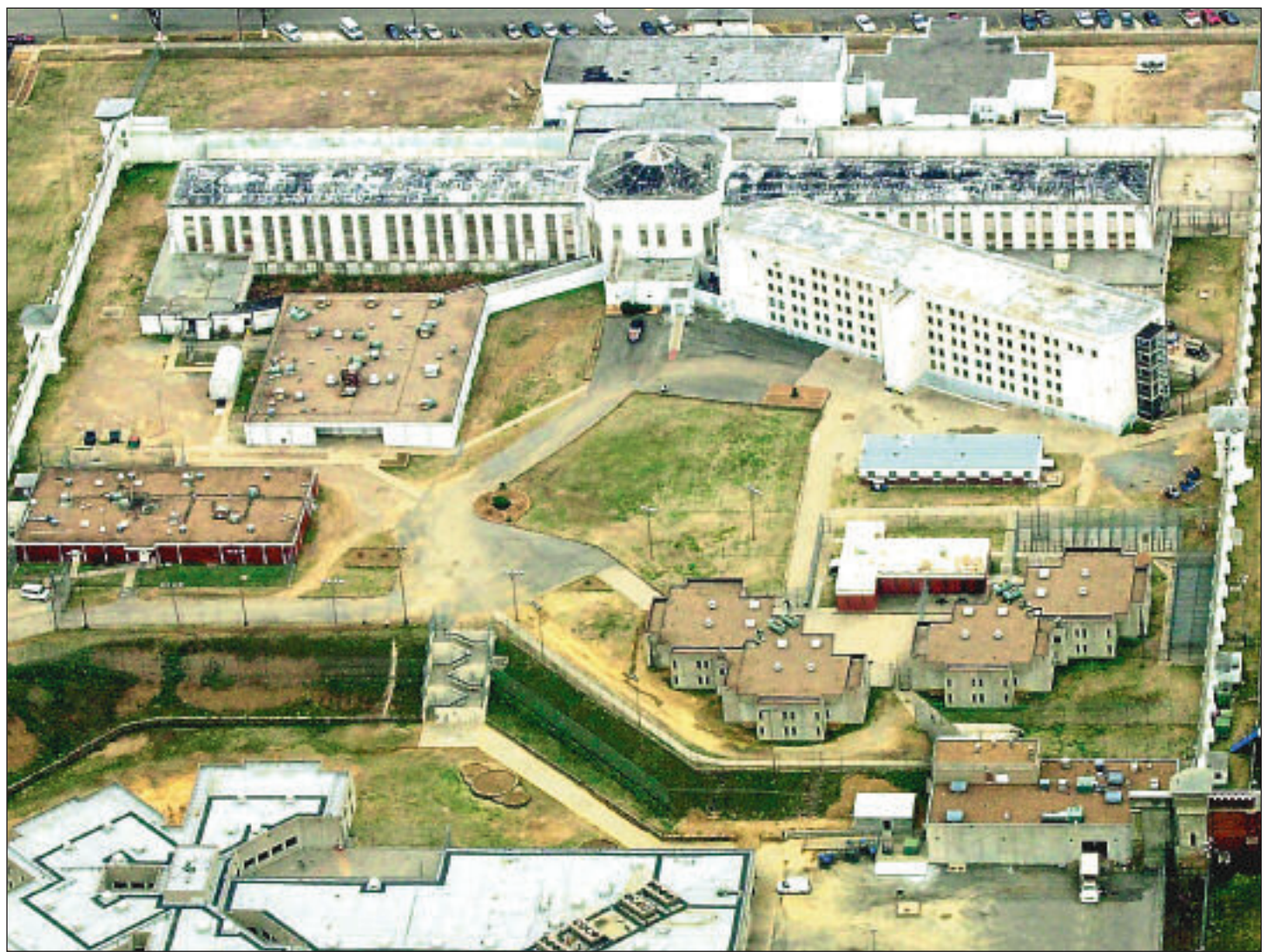
A preliminary architectural and engineering study of state correctional facilities showed nine of the 30 buildings that make up the Oklahoma State Penitentiary at McAlester need major repairs, major renovations or to be torn down. TOM GILBERT/Tulsa World
